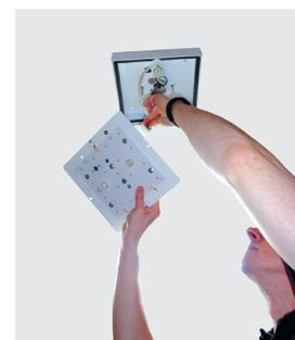
6. Connect new gear tray to slip plug.
