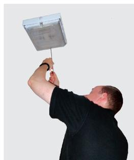
1. Isolate fitting and unscrew diffuser.
