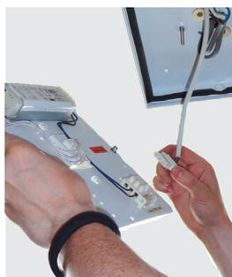
5. Unplug slip-plug and remove gear tray.
