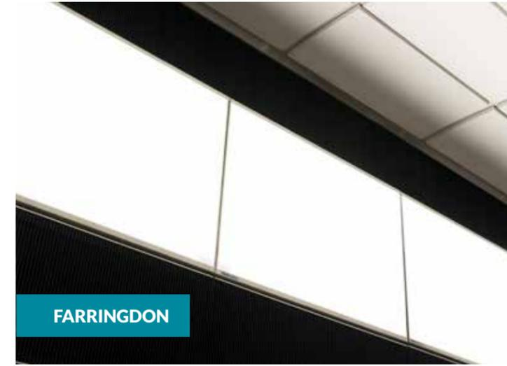
“The regulations affecting all luminaires specified by Crossrail, are contained in a document practically an inch thick” explains James. “Accordingly all our light boxes are designed in accordance with the Fire Precautions (Subsurface Railway Stations - England) Regulations 2009, commonly known as section 12, and comply with London Underground’s subsurface standard 1-085.
