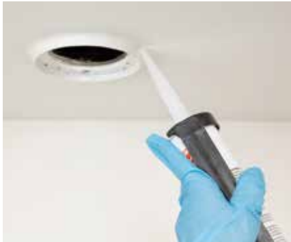
1. Fit mounting bezel & apply anti-pick mastic
